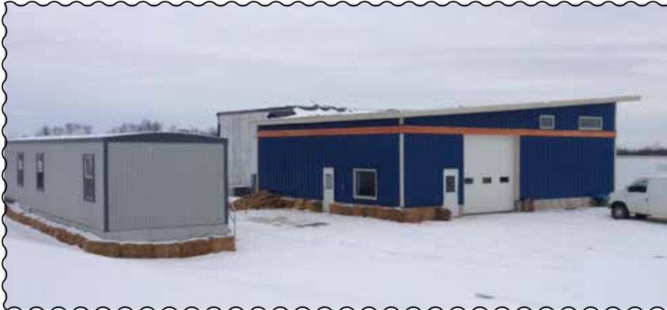
Our new packing shed (center) with the office & crew trailer on the left and big walk-in cooler poking up behind.
